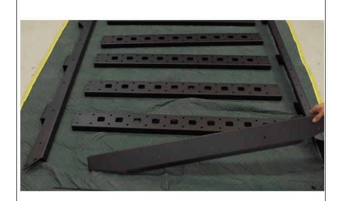
14. Bolt rest of rack together with M6x25 button head cap screws, washers and flange nuts.
